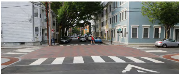
▲ A raised intersection with well marked crossings keep motorist speeds to 20 mph 24 hr a day in Cambridge, MA.
