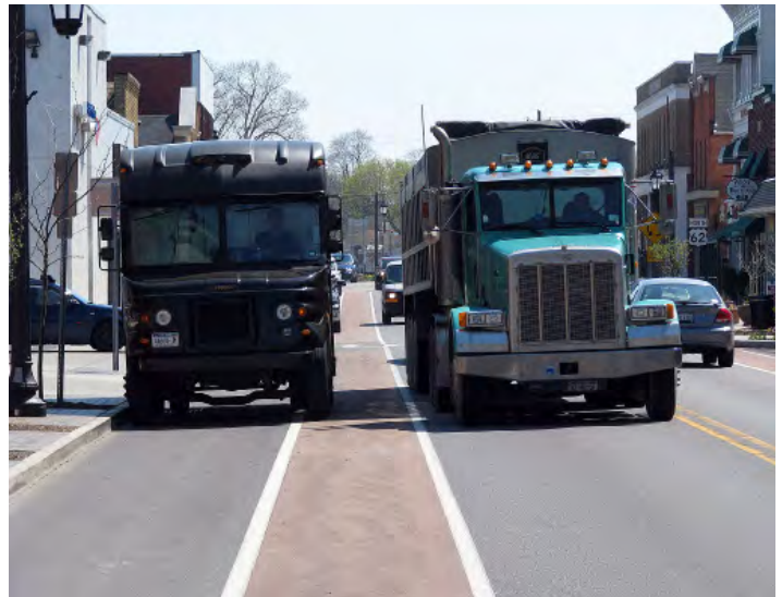
▲ Route 62, Hamburg, NY vehicle lanes are made narrow and colorized “door-zone” to help separate moving vehicles from people entering a parked car. Route 62 is a major truck route for the State of New York.
